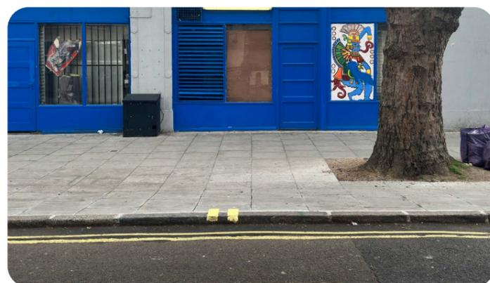
To support better environmental practices, the existing paving slabs on the pavements (left) will be cleaned and reused where possible for most of the project.
