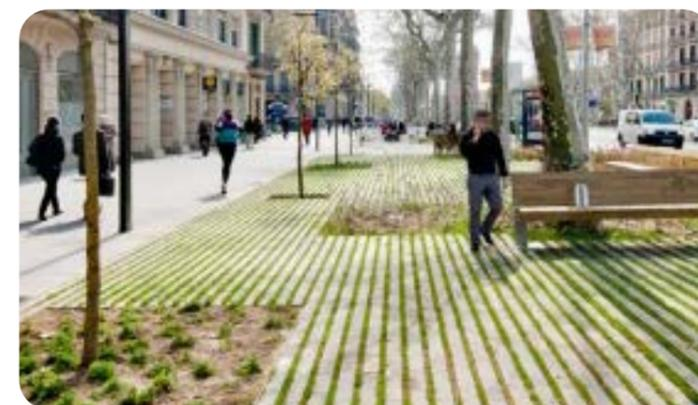
Grasscrete is created using paving blocks through which grasses can grow. This creates a firm and accessible surface for wheelchair users and buggies, but creates a softer feel than asphalt. It is also permeable, helping to manage storm water run off.
