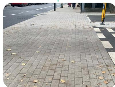
Informal crossing points or continuous crossings can be used on each side of the junction to create a continuous walking route and make it clearer that drivers need to give way
