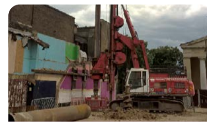
Continuous bored piling
