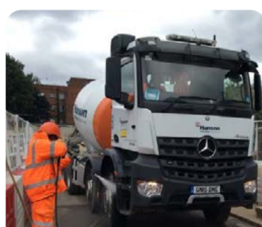
Jet washing vehicles on-site
