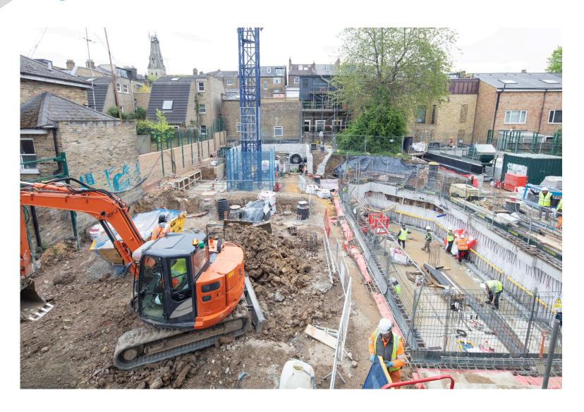
**Substructure and Foundation:** Basement Reduced Level Dig Complete, Ground Floor Slab Pours are now on going. Deep drainage works and attenuation tank complete.
