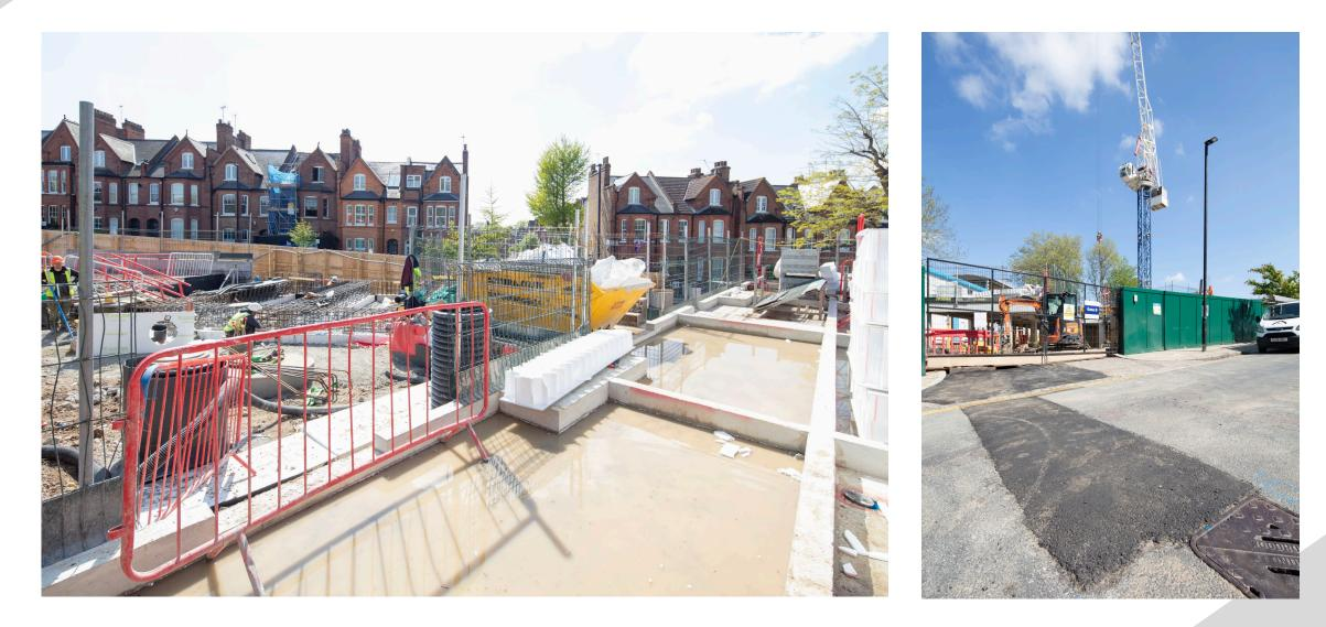
**Substructure and Foundation Construction:** Block C and Block A Foundations are nearing completion with the Ground Floor Slabs and Lower Ground Floor Slabs now poured. Block B is working in line with our programme, preparing for the Ground Floor Slab pour.
