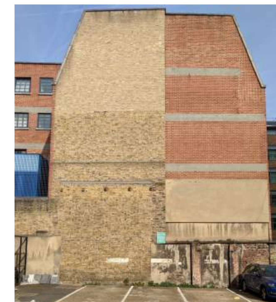
Existing flank wall near Devonshire
