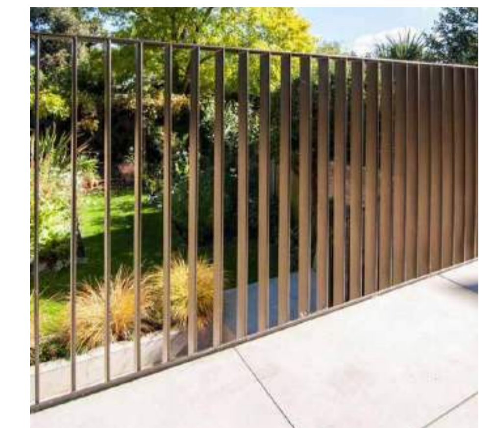
1.5 high balustrade fencing
