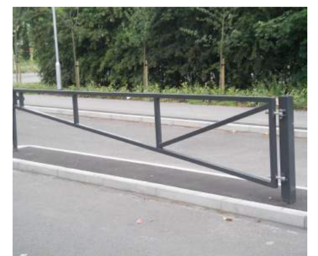
Vehicle stopping gates
