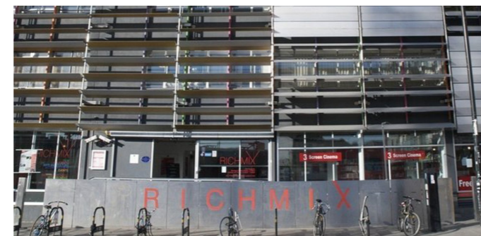
Community and cultural building, Rich Mix
