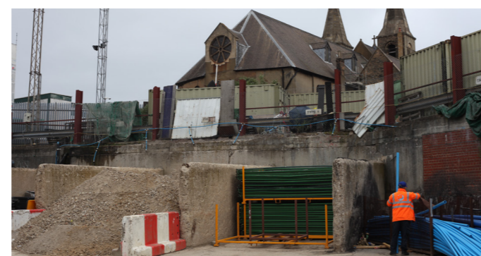
Significant level changes
