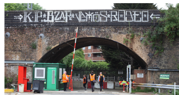
Constrained access into area
