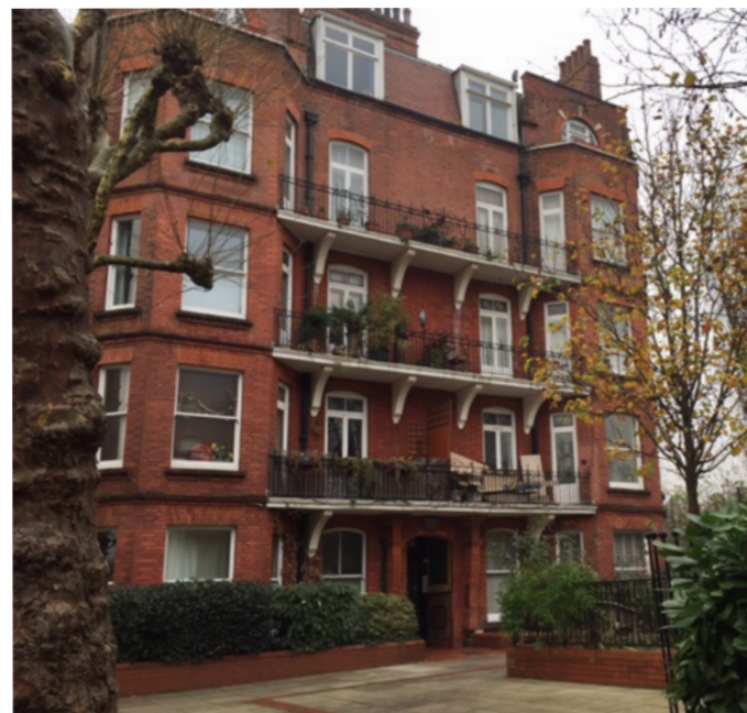
Mansion blocks, Lissenden Gardens
