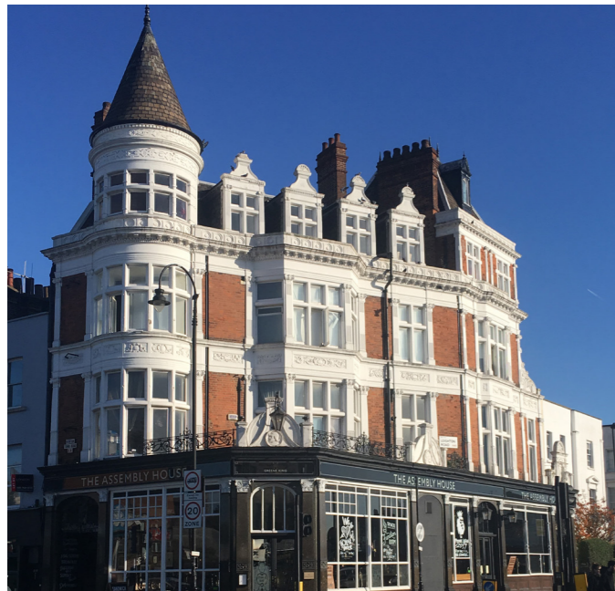
Articulated roof form, Assembly House, Kentish Town Rd
