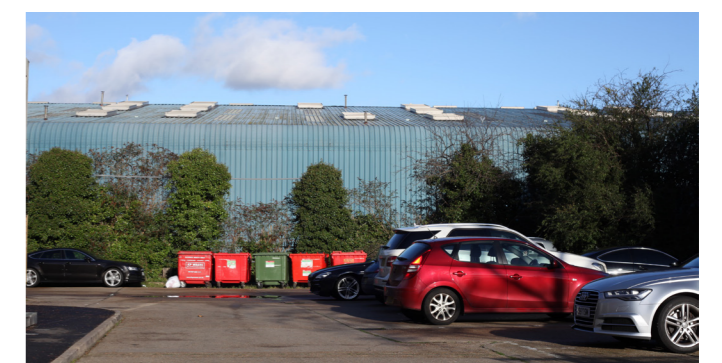
Poor quality buildings and public realm
