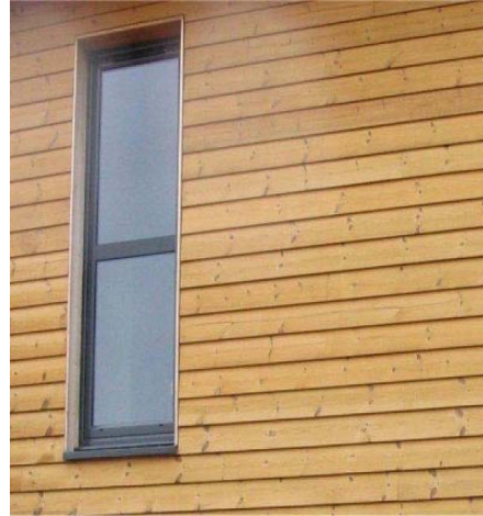
Timber clad finish on external wall insulation
