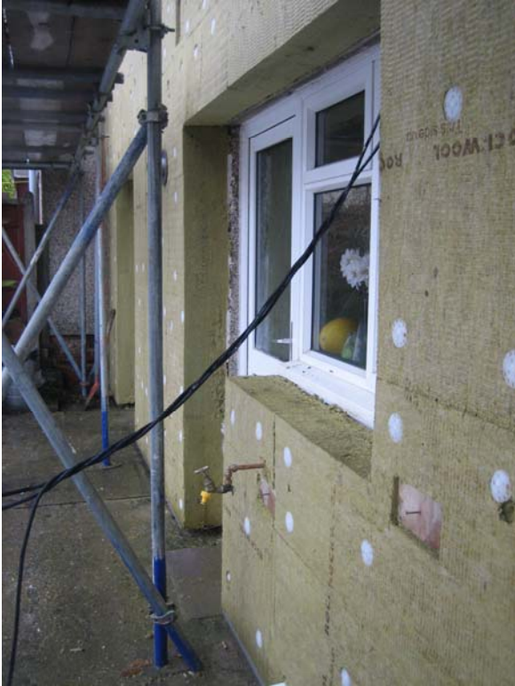
Installing external wall insulation Picture Credit: ECD Architects
