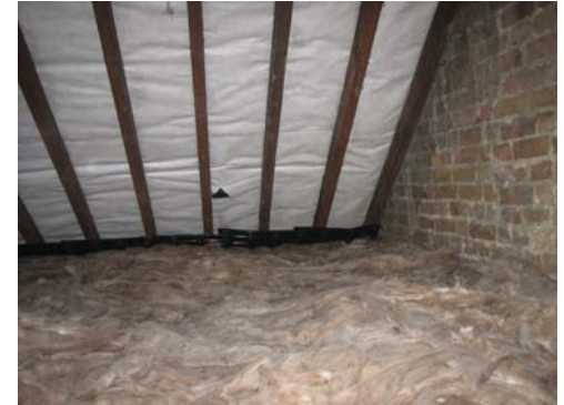
Insulation installed between and over joists in loft. Picture credit: ECD Architects
