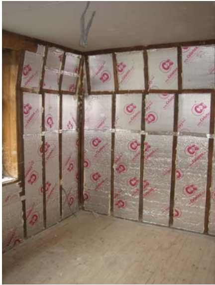
Internal Wall Insulation Picture credit: ECD Architects
