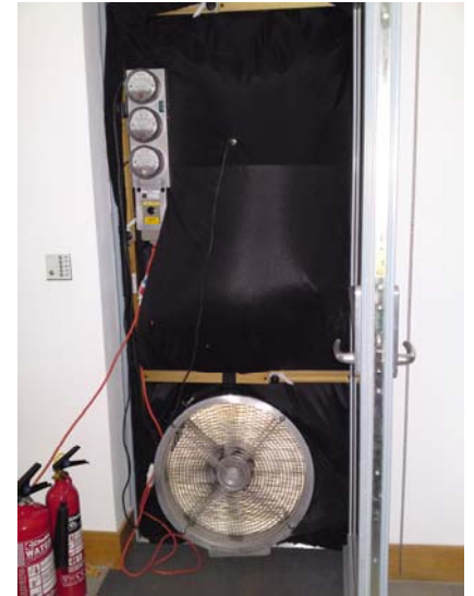
Fan pressurisation test equipment set up Picture credit: ECD Architects
