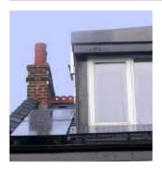
Solar photovoltaic (PV) panels can be used to generate electricity from sunlight. Panels are usually roof-mounted, and should be oriented southwards and be tilted between 200 and 500 from the horizontal. Solar slates or tiles are also available, for use where maintaining the original appearance of the roof is important. Solar slates and tiles are currently double the price of panels (2012) but are expected to fall to a comparable price by 2020.
