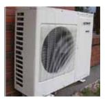
A heat pump works by extracting heat from an external source and supplying it to the property for heating or domestic hot water. Heat can be extracted from the ground, from water or from the air.
