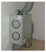
Whole house MVHR systems run continuously, extracting moist stale, air from kitchens and bathrooms, and supplying fresh air to living spaces and bedrooms, via ducts. The systems recover some of the heat from the extracted air and use it pre-heats the incoming fresh air. Modern MVHR systems use energy efficient DC fan motors for low fan power, and incorporate plastic cross-flow heat exchangers to achieve heat recovery efficiencies as high as 90%.
