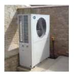
Air source heat pumps need to be situated where they will get a sufficient flow of air and the optimum location is likely to be freestanding in a rear garden. You are advised to consider the location and colour of the unit so that it blends in it with a garden setting and so that the visual impact is minimised, A noise impact statement will be required with a planning application for an air source heat pump.
