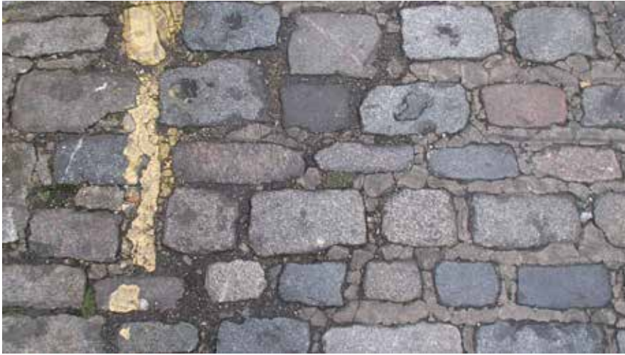
Poorly bonded granite setts, Bleeding Heart Yard
