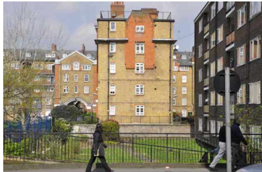
Bourne Estate viewed from Baldwins Gardens
