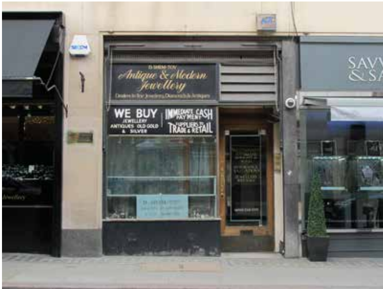
88-90 Hatton Garden (ii, facing Greville Street)
