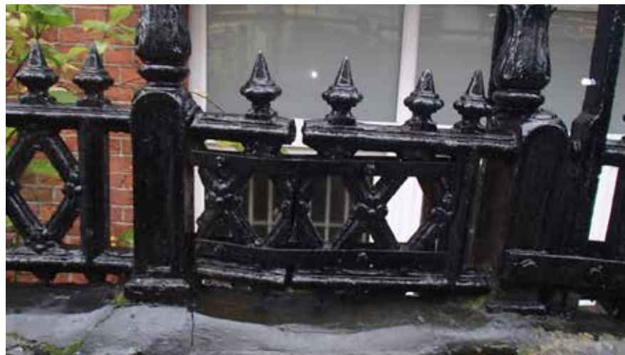
Damaged railing, 59-61 Hatton Garden
