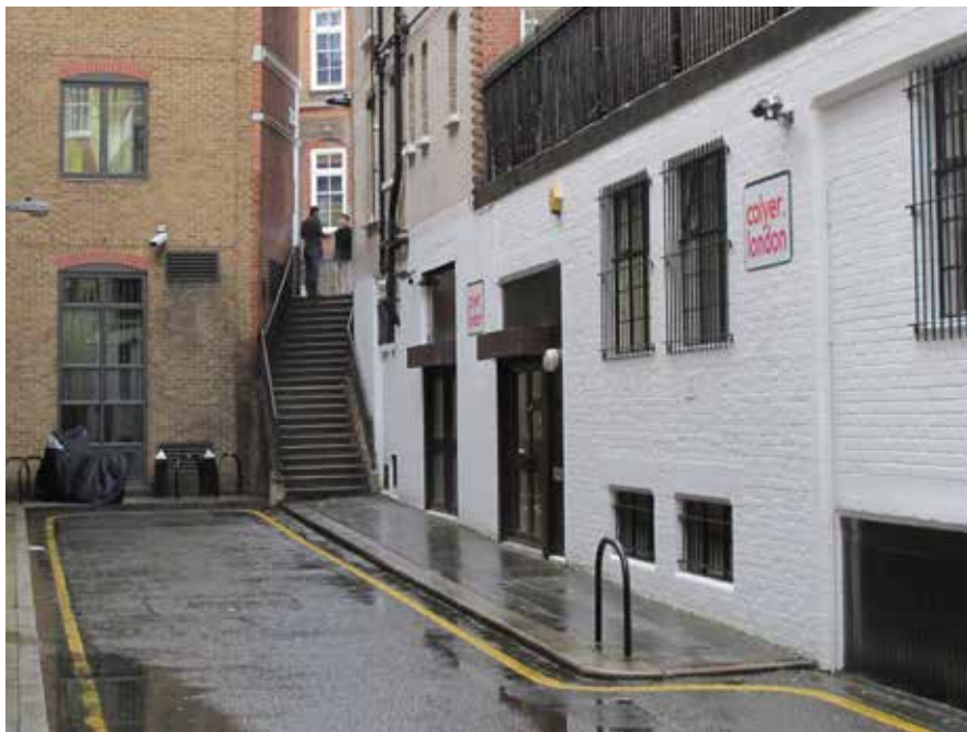
Painted brickwork, Vine Hill
