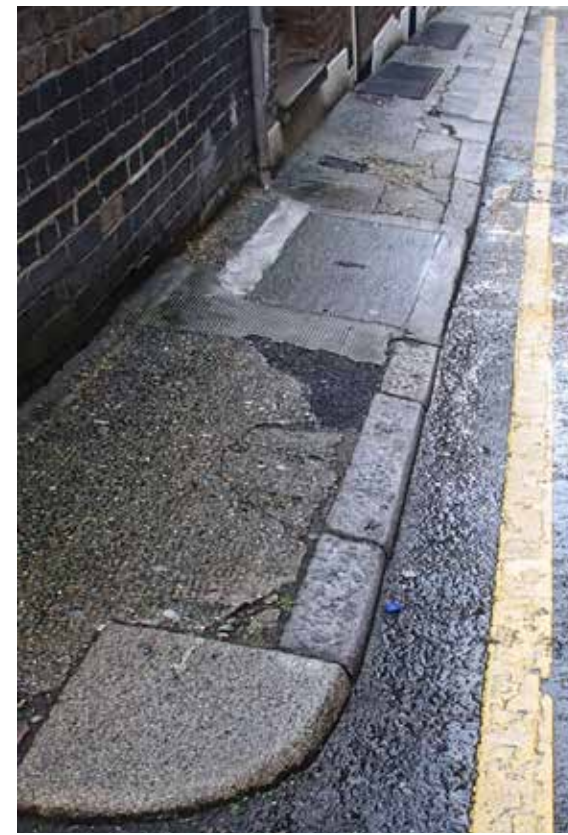
Poor-quality paving, Vine Hill
