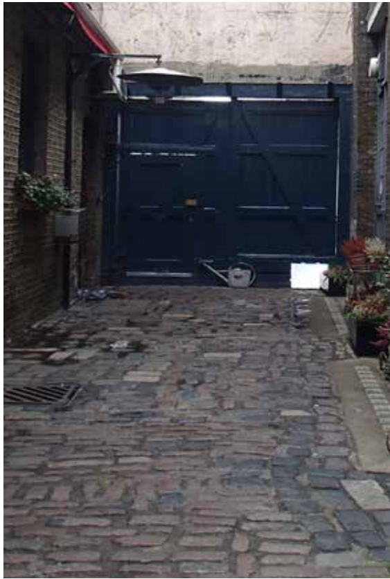
Badly re-laid granite setts, Bleeding Heart Yard
