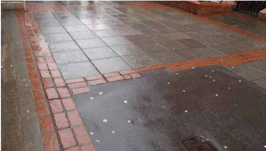
Damaged paving, Leather Lane by Waterhouse Square
