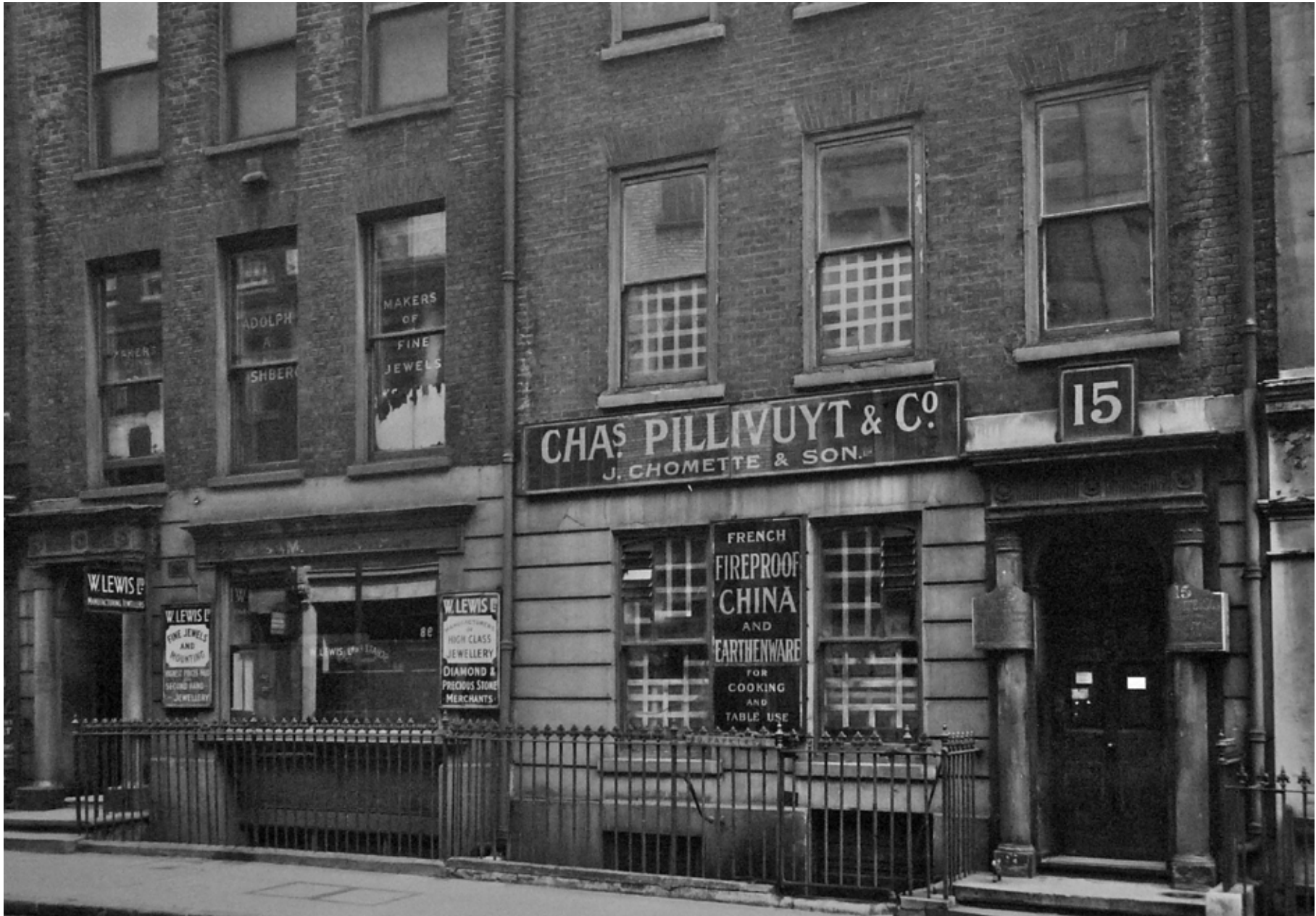
Georgian houses at 15 and 16 Hatton Garden, photographed in 1944 and demolished c. 1970s (LMA)
