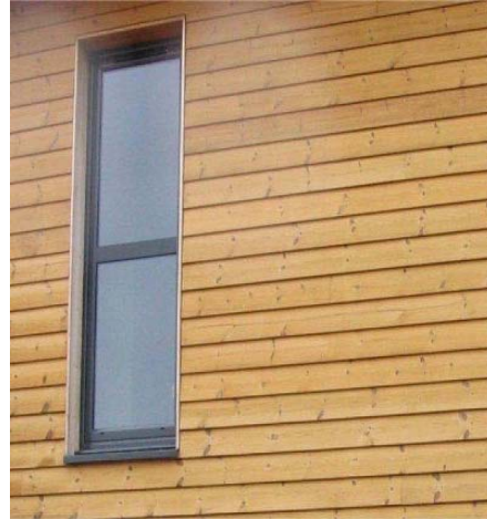
Timber clad finish on external wall insulation
