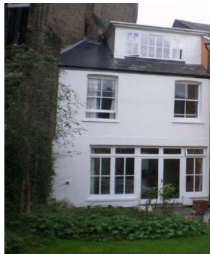
Render finish on external wall insulation Picture credit: www.victor.co.uk
