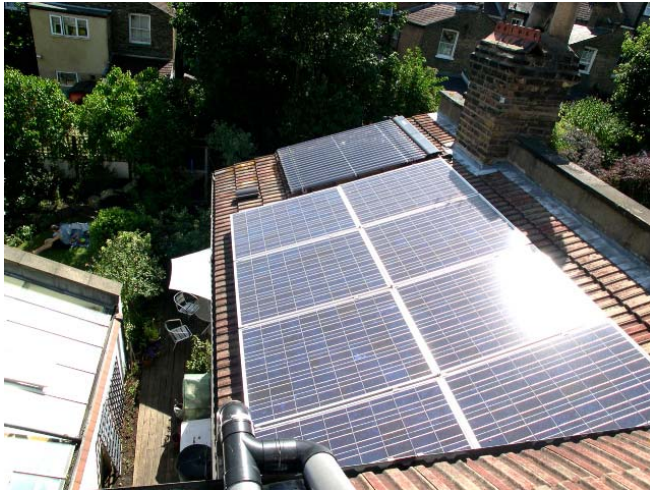
Solar thermal (hot water) panel (top) next to photovoltaic (PV) panels Picture credit: www.victori.co.uk
