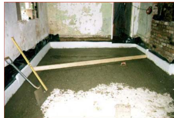
Insulation of a concrete floor. Picture credit: John Willoughby
