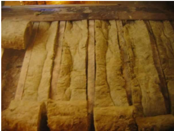
Insulation of a timber floor. Picture credit: John Willoughby
