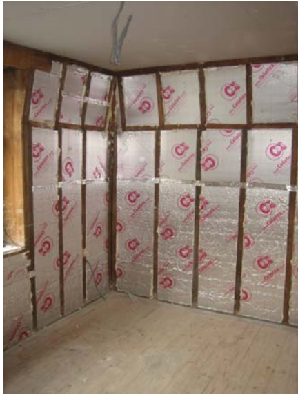
Internal Wall Insulation Picture credit: ECD Architects
