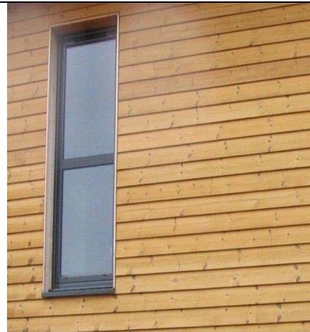
PHOTO 3 – Timber cladding
