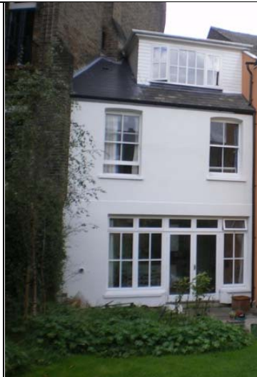
PHOTO 2 – After external wall insulation
