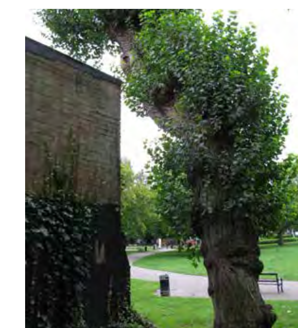
Proximity to building
