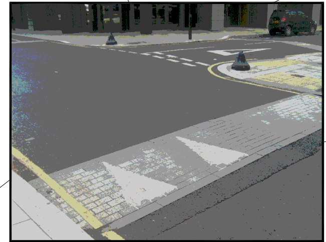
This photograph shows a typical raised junction
