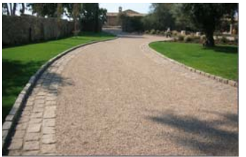
'Tar spray and chip' as alternative surface finish
