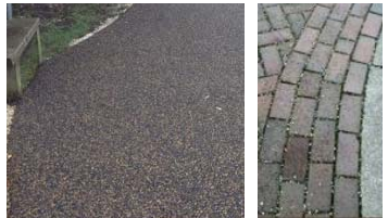
Recycled rubber and stone porous paving system and stone edging
