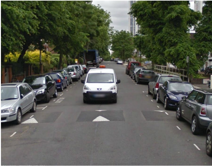
Existing speed cushions on Fellows Road
