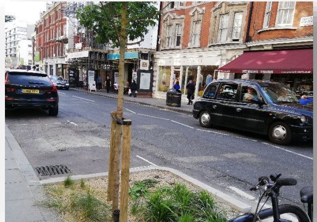
A tree in a pavement build-out/extension
