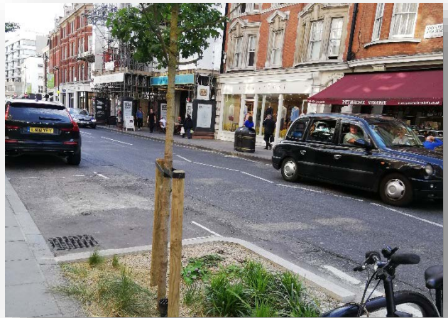
A tree in a pavement build-out/extension
