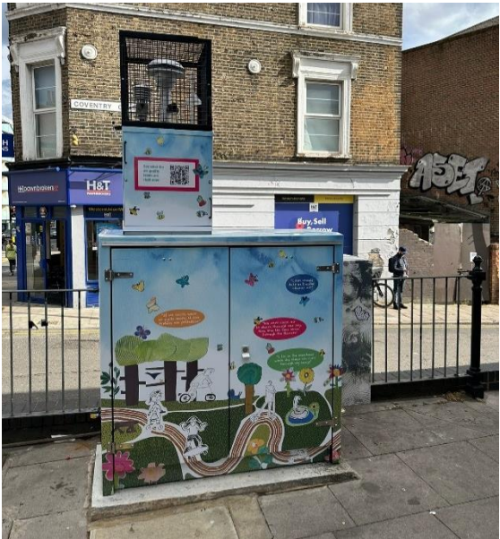
Figure 8 (right): An automatic monitor on Kilburn High Road. This one was installed in 2026 and measures nitrogen dioxide (NO 2 ), coarse particulate matter (PM 10 ), fine particulate matter (PM 2.5 ), and ozone (O 3 ).
