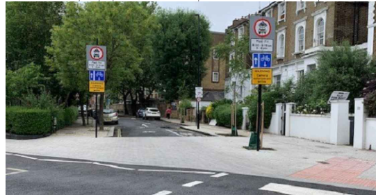
Example of a continuous footway in Camden
