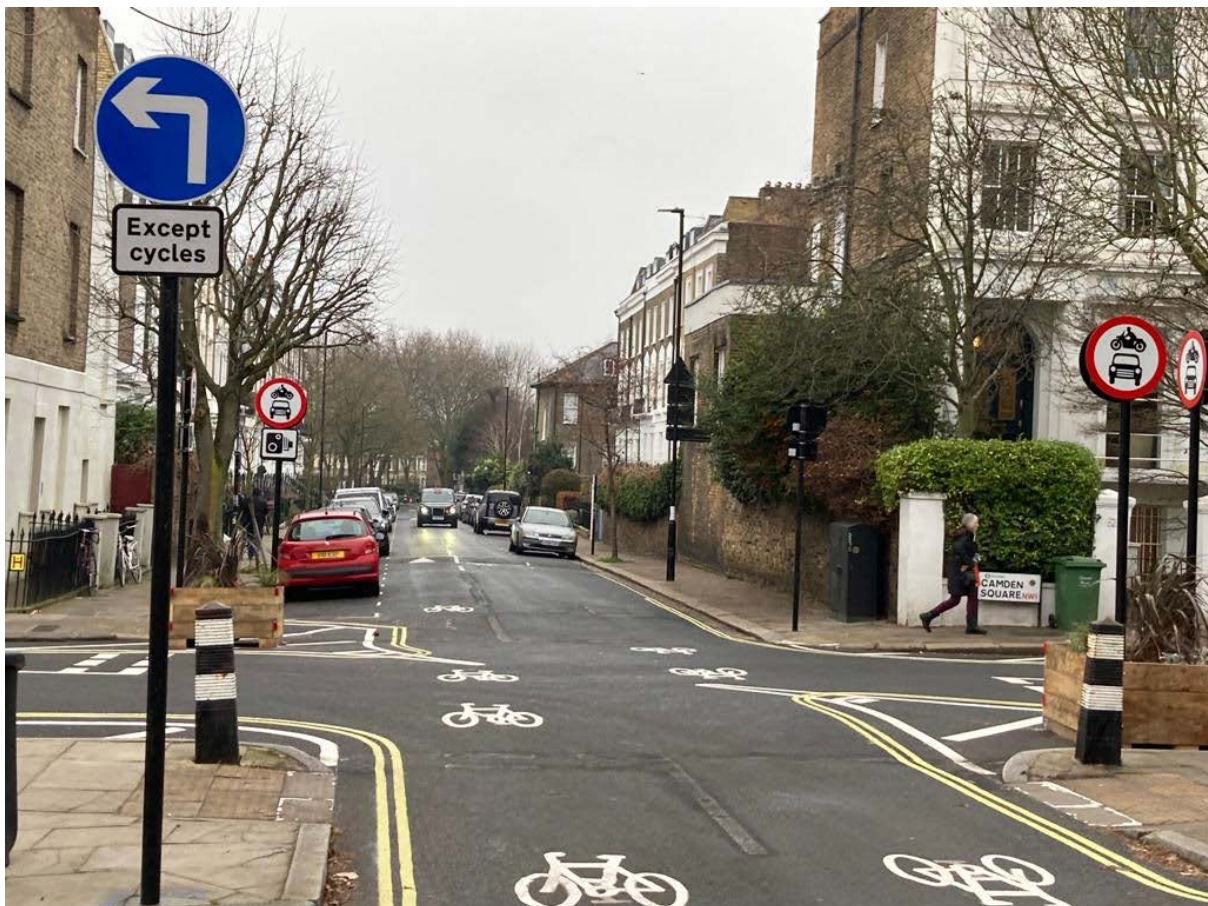
Image shows diagonal motor vehicle restriction at junction of Camden Square, Murray Street and Stratford Villas with a taxi approaching along Stratford Villas
