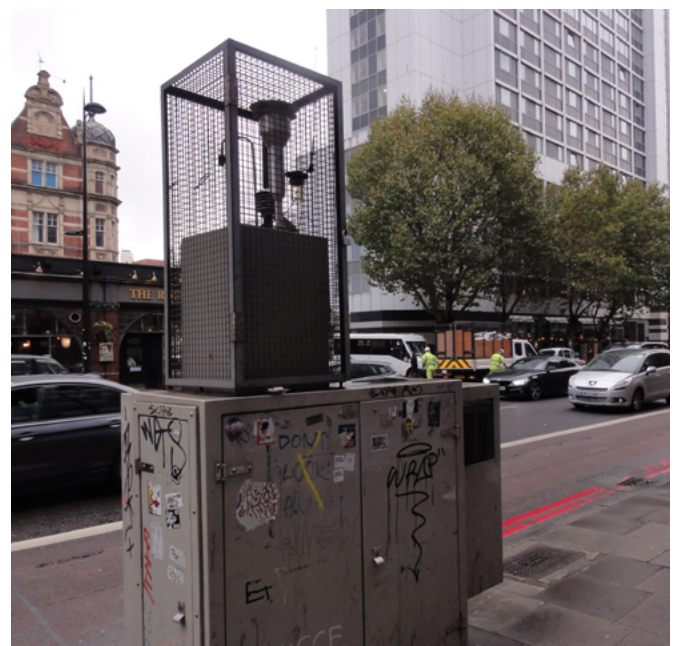
AIR QUALITY MONITORING STATION ON EUSTON ROAD
