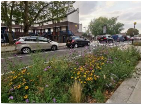
Rain garden on footway
