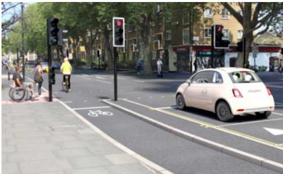
Figure 3.9: Separate cycle signals at junctions
