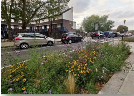
Rain garden on footway
