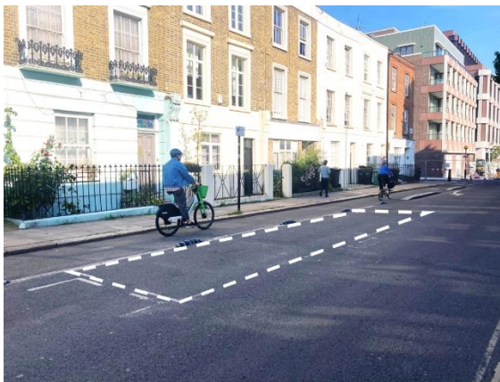
Floating loading bay between cycle lane and carriageway
