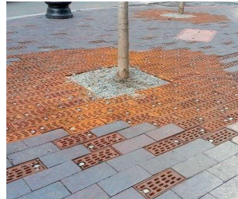
Hard surfaces should play a role in a sustainable drainage strategy where possible
