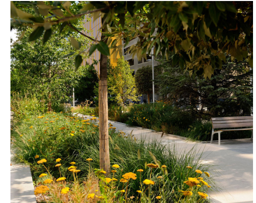
Innovative water management wherever possible (SuDS and permeable paving)
