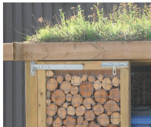
Urban greening including green walls and bin stores with green roofs should be explored
