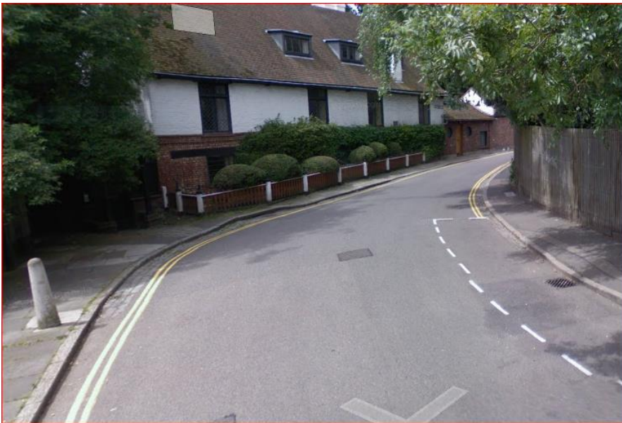
Millfield Lane: narrow pavements make it difficult for pedestrians to use the street safely
