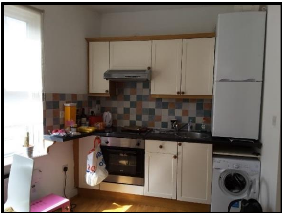
Inappropriate stacking of floor standing fridge freezer above washing machine
