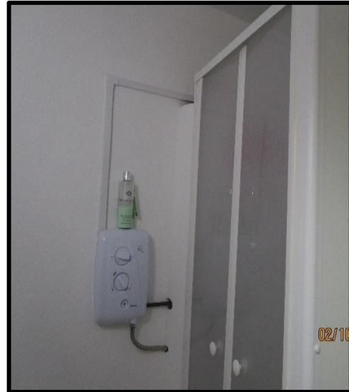
Shower mixer controls located outside of shower cubicle + dangerous wiring
