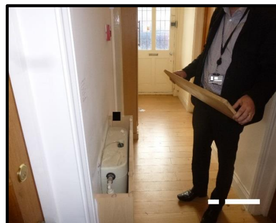
WC cistern for flat located in common parts due to space limitations, resulting in breach of fire separation of wall
