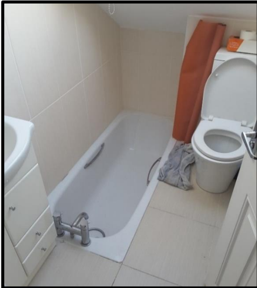
Sunken bath with restricted headroom and smooth floor tiles. Likely to result in trips/falls
